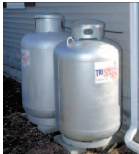
FIGURE 4-3 Simple residential and commercial propane installation.
