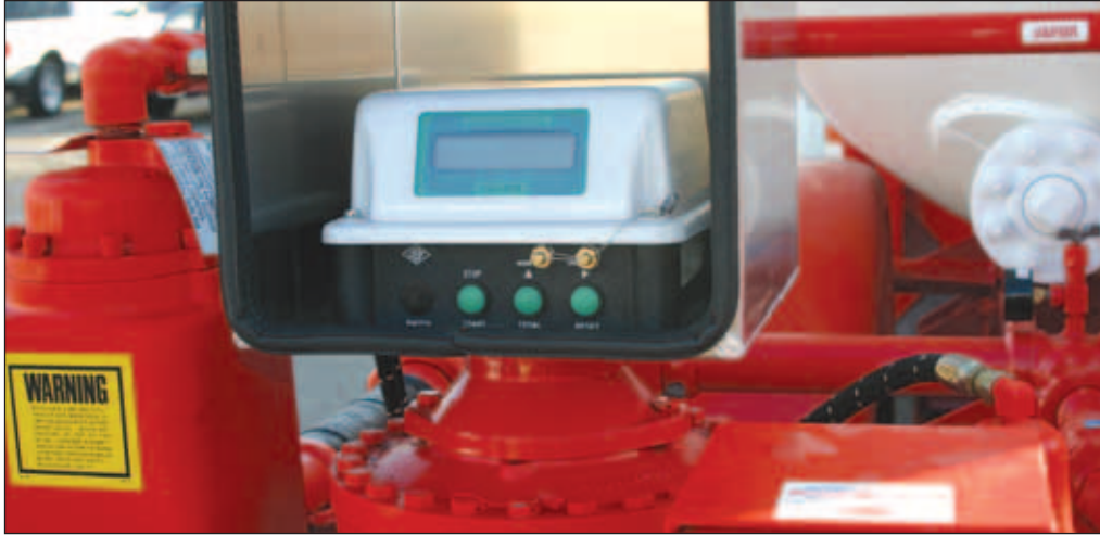
FIGURE 5-9 OFF-truck remote shut-off device.
