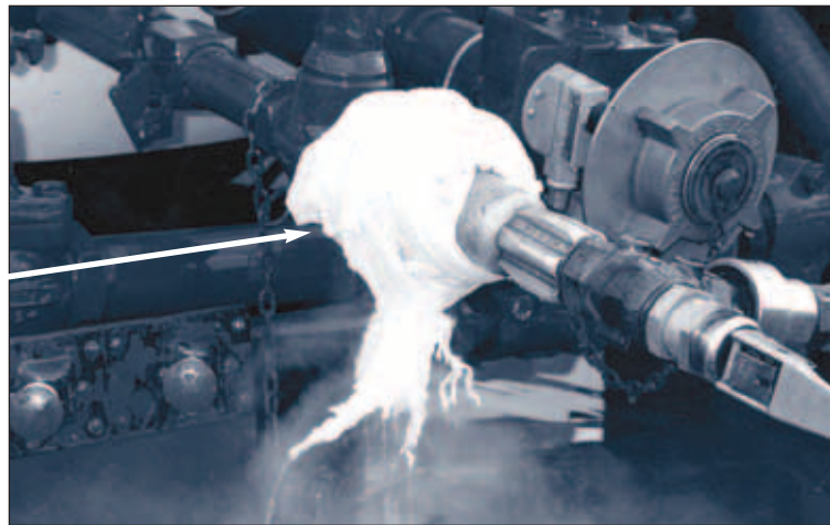
FIGURE 8-21B Liquid leaks may be controlled by freeze wrap.
