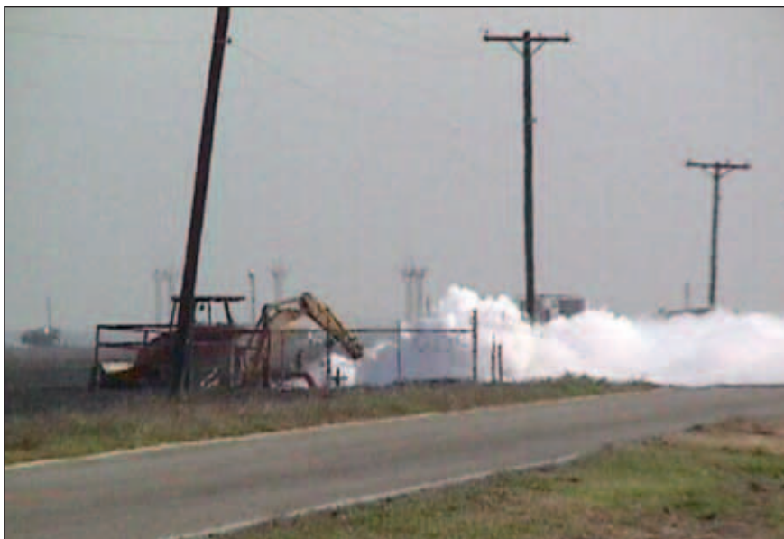
FIGURE 7-2 Incident involving a propane pipeline that was struck during excavation operations. Firefighters initiated non-intervention operations given the remote location of the incident and the need to shutdown the pipeline.
